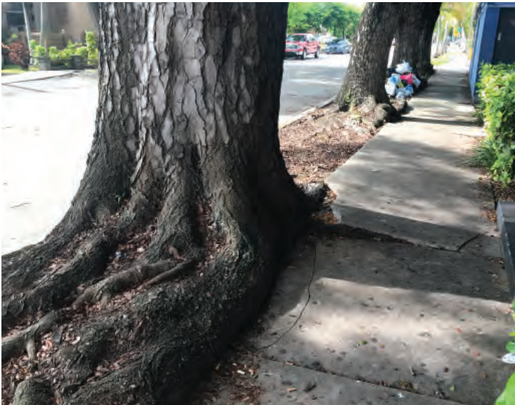
Above: Mahogany trees in La Pastorita that have outgrown their space. This is an extra large species planted in a 3-FT swale (should be at least 15FT).
