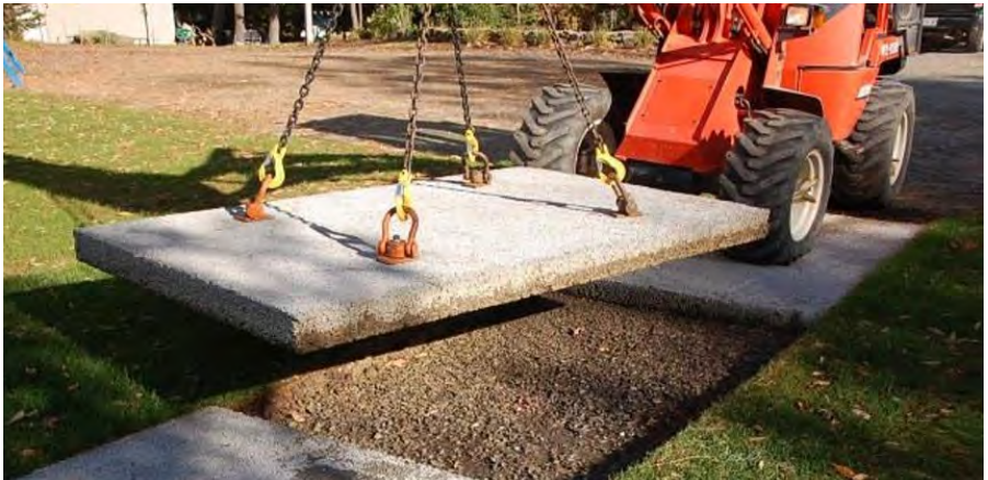
Precast porous concrete sidewalk and installation photo. Source: Stormcrete, Porous Technologies, LLC
