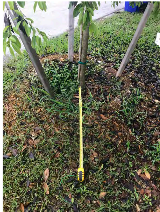
Inspection of tree installation in Douglas Park revealed that the planting hole was barely larger than the rootball, less than 3’ radius
