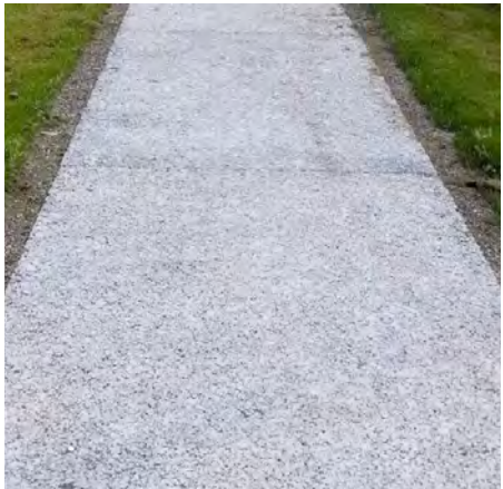
Precast porous concrete sidewalk and installation photo. Source: Stormcrete, Porous Technologies, LLC
