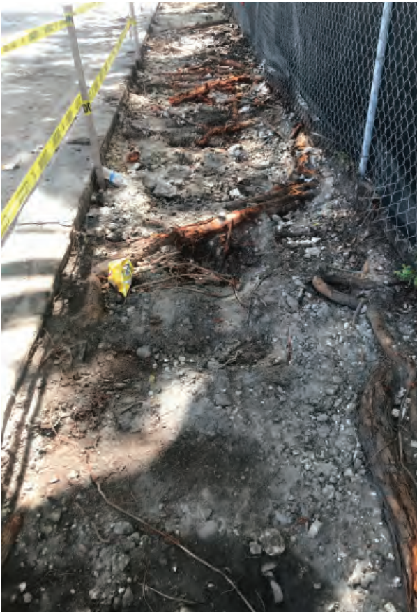
Above: Mahogany trees in La Pastorita that have outgrown their space. This is an extra large species planted in a 3-FT swale (should be at least 15FT).
