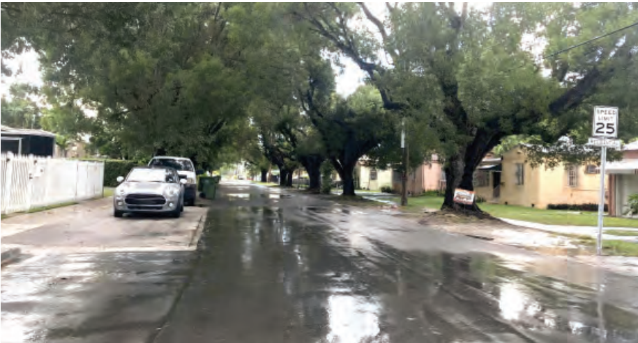
Pervious concrete swale in Parkdale South on left is dry during rain event - dirt swale on right is puddled from compaction due to cars.
