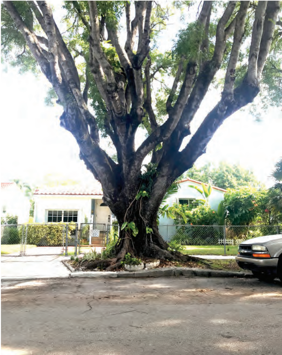
Large mahogany tree in Shenandoah that has cracked the curb and the adjacent road.
