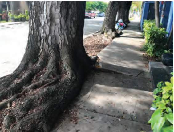
This thin planting strip was not the appropriate place for this large species tree which is now heaving the sidewalk
