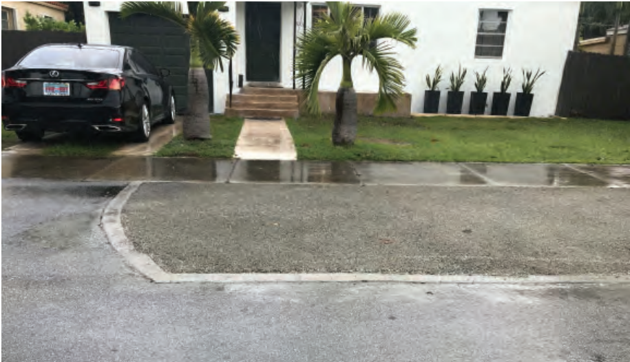
Pervious concrete swale in Parkdale South
