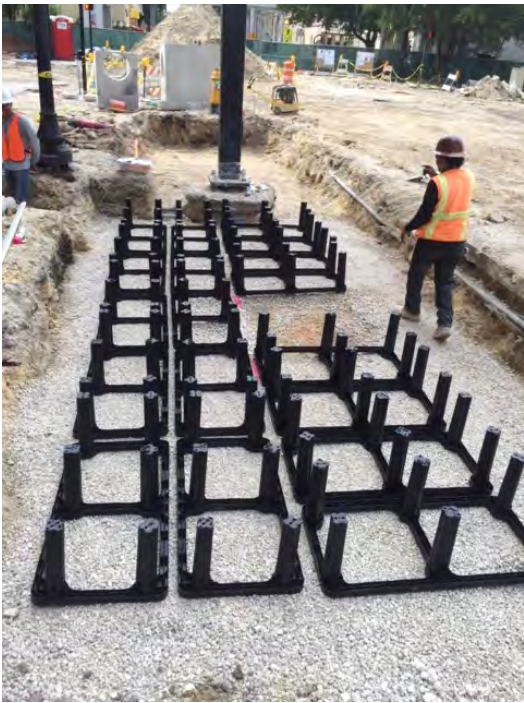
Silva Cell Installation on Flagler Street, Miami 2018
